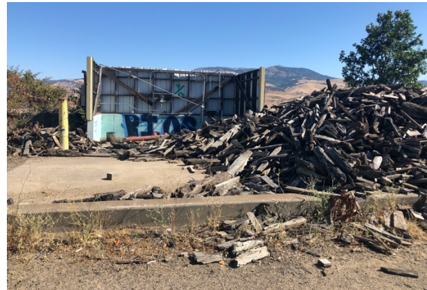
Former mill structures at center of site
